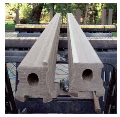
Figure 1. Stock pieces of EverGrain Designer Universal Rail form the frame for the author's vertical-rod railings. So he can use deck boards for the cap rail, he has removed the ridge from what will be the upper rail (right in photo), with a circular saw.
