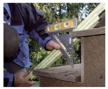
Figure 4. Holes in stair rails have to be drilled at the correct angle, which is easily measured using a level and a Speed Square (left). To make a drill guide (below) for the stair rails, the author drills through a scrap of decking and cuts it in half along the drill hole. He then cuts the bottom of the scrap to the angle he measured above.
