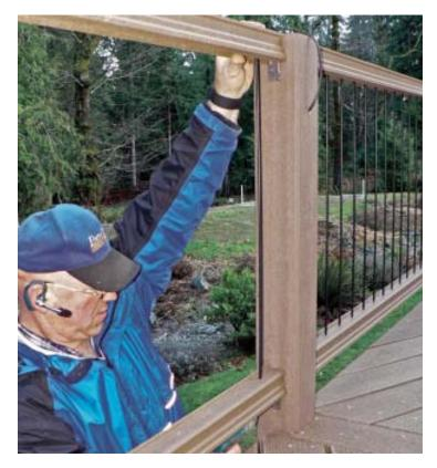
Figure 3. After installing the top rail, rods precut to the correct length help determine the bottom rail's height. With the rod bottomed out in the lower rail, the author raises the rail until he feels the rod become flush with the top of the upper rail. That's when he screws home the lower rail's support bracket.
