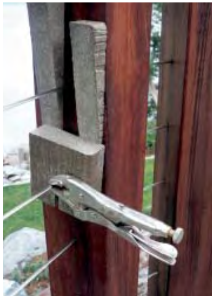
Figure 14. Snug up the cable before final tightening. Locking pliers gently closed on the cable provide the grip. Wedges provide the force to stretch the cable. Stretch from several spots along the run, particularly at corners.
