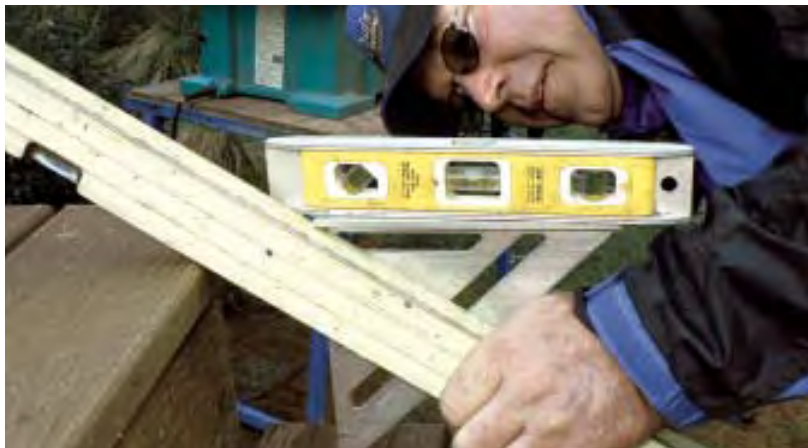
Figure 12. Tools you probably already own determine the angle for drilling the stair posts. A long level on the tread noses establishes the stair pitch, and a Speed Square, held level, measures the angle.
