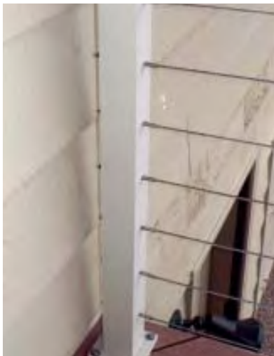
Figure 5. Space end posts from the house to leave room for a wrench to tighten the cables.
