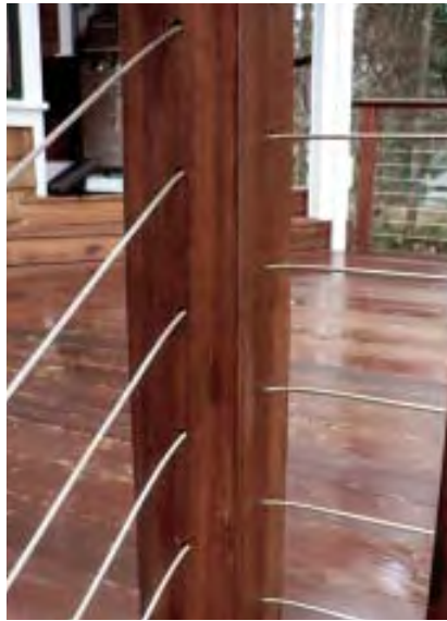
Figure 3. When a cable has to turn a corner at a single post (left), one method is to drill a curved hole through the post (A). Because there's a lot of tension on the inside corner of these posts, hardwood such as ipe is recommended over soft cedar or pine. The second way around a single-post corner is for two cables to terminate at that post (B). For the cables to run at the same level, the hole for one cable stud must be angled to miss the other stud (C).
